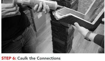
The caulking should seep from the top of the connection when placed around the post.
