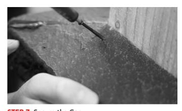
**STEP 7: Secure the Cap** Insert two screws diagonally into each side of the cap connecting the cap to the post.
