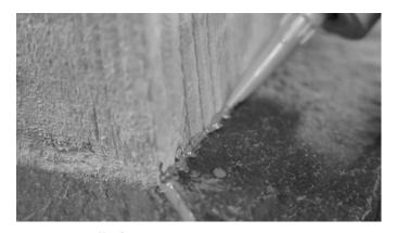
**STEP 8: Caulk the Connection** Run a bead of GenStone eXact Color caulking in the void between the cap and the post on all sides.
