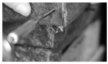
**STEP 7:** Connect the Cap Carefully insert one screw in each connection and cover the screw with GenStone eXact Color caulking.
