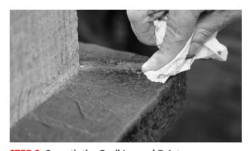
**STEP 9: Smooth the Caulking and Paint** Using a glove or paper towel, smooth the caulking and wait for the caulk to dry before painting.
